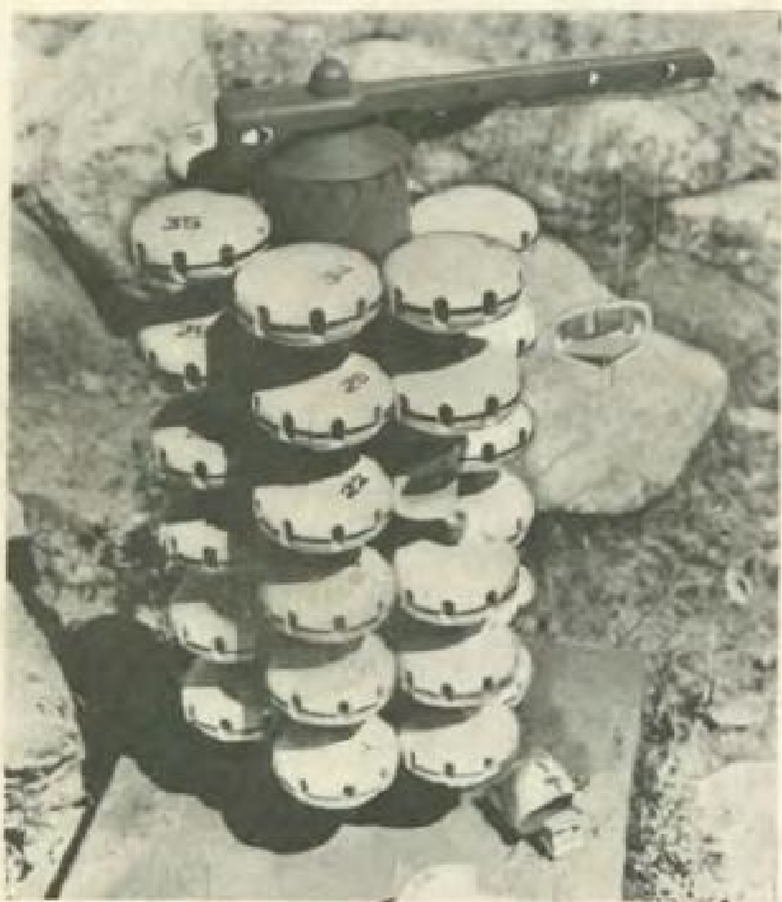
Mobil space residential unit — a dwelling for shepherds, builders, geologists et etc, is formed of telescopic sector folds. Author of the project — architect Saken Narinov, Alma-Ata.
