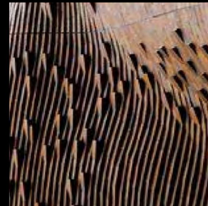
Examples of sound diffusive profiles
